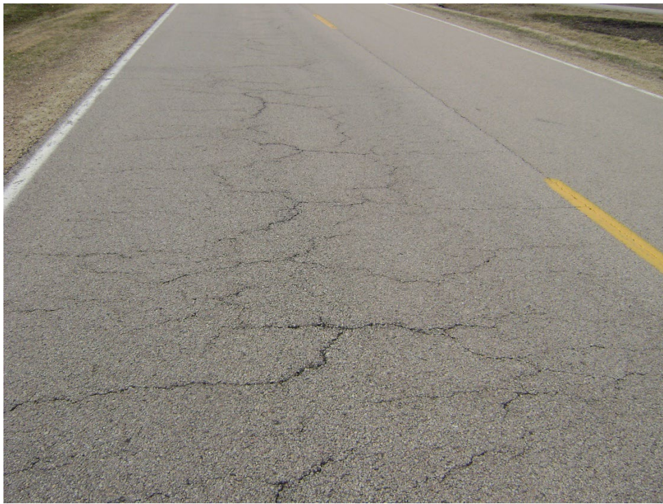
Asphalt Rating 4 – Fair, irregular shaped block cracking over 50% of pavement
