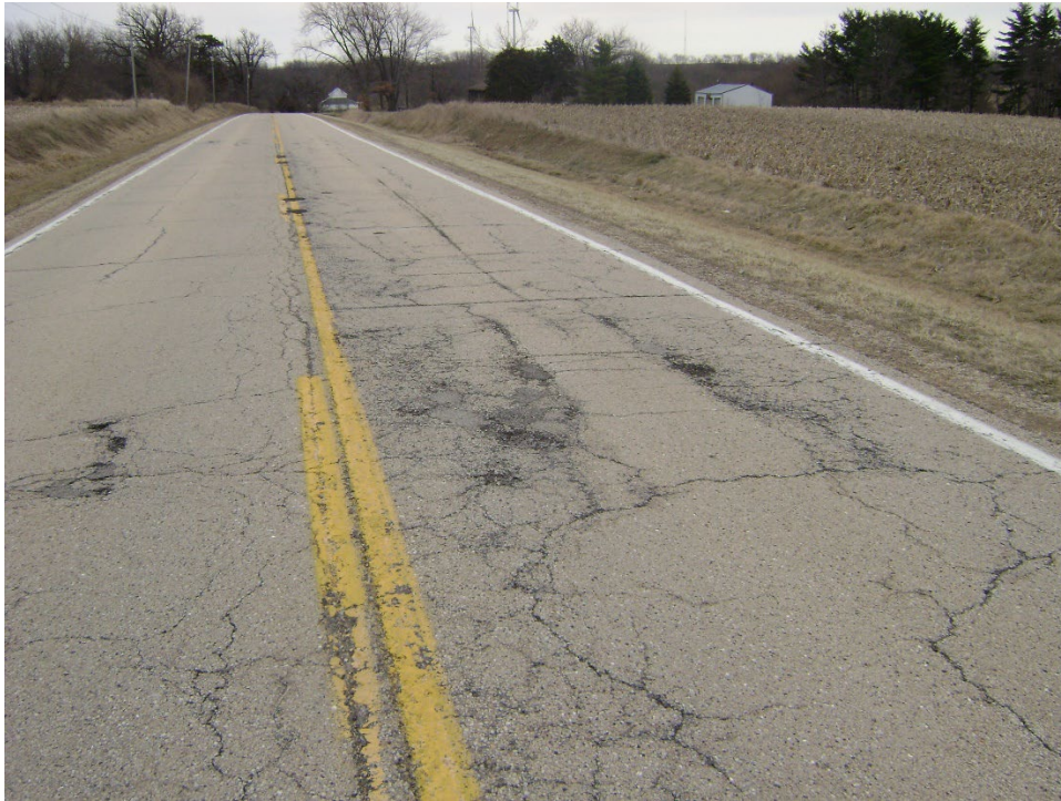
Asphalt Rating 3 – Poor, alligator cracking and potholes beginning
