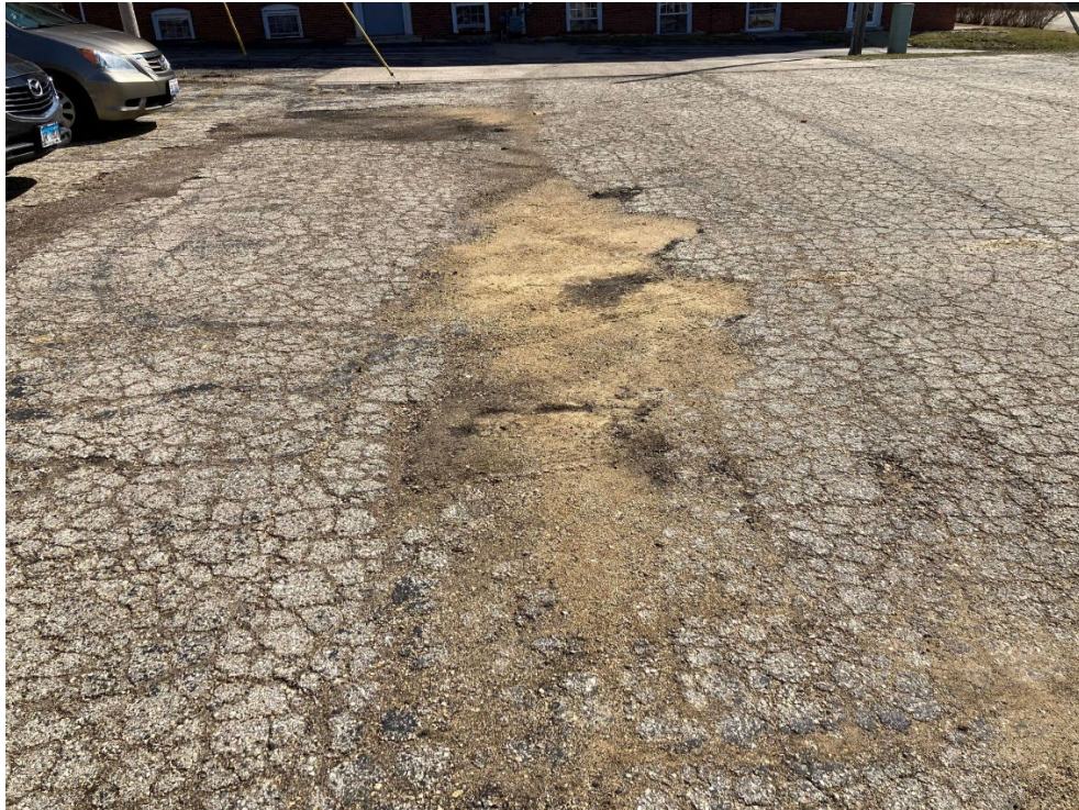
Asphalt Rating 1 – Failed, surface has lost its structural integrity
