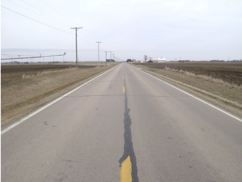
Asphalt Rating 7 – Good, transverse cracks more than 10 feet apart with crack filler
