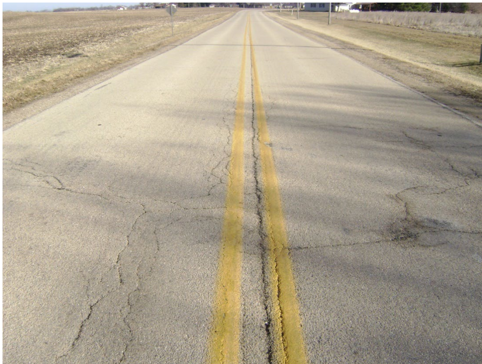
Sealcoat Rating 3 – Fair – cracking throughout sealcoat
