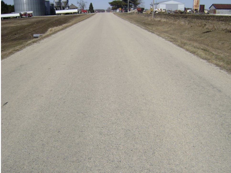
Sealcoat Rating 4 – Good – some aggregate loss
