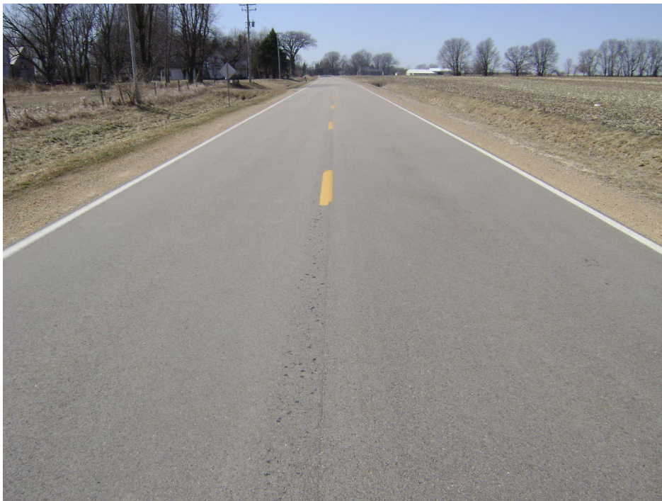
Asphalt Rating 8 – Very good, no issues of concern
