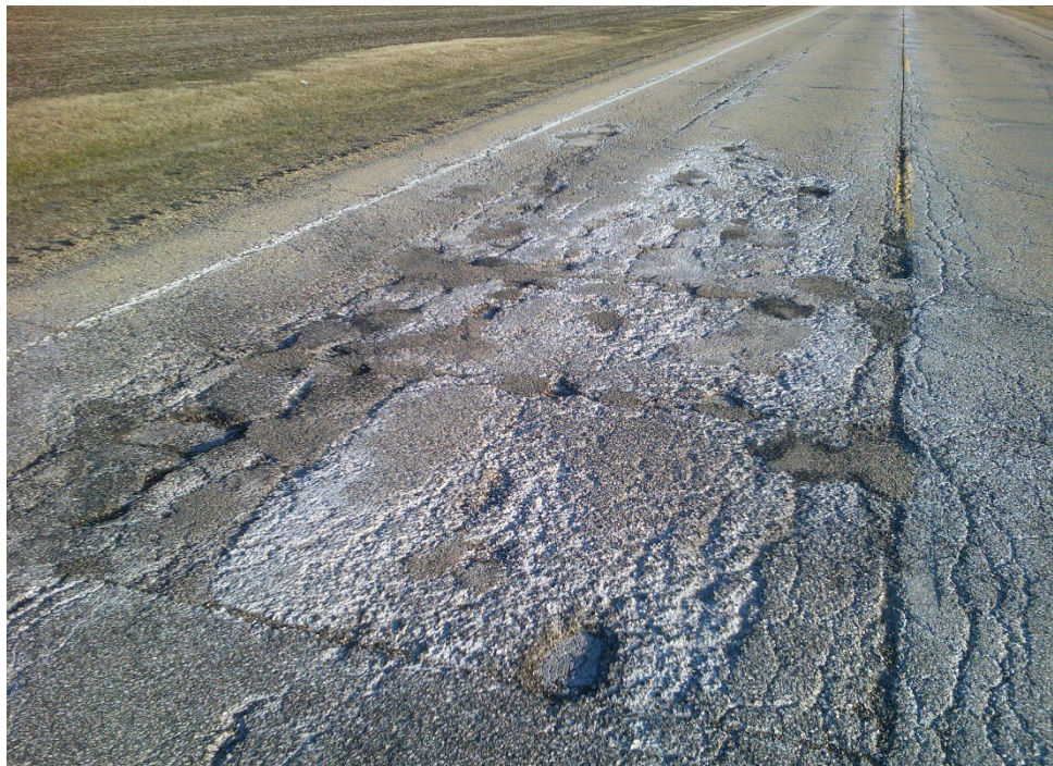
Asphalt Rating 2 – Very Poor, potholes and patching in poor condition
