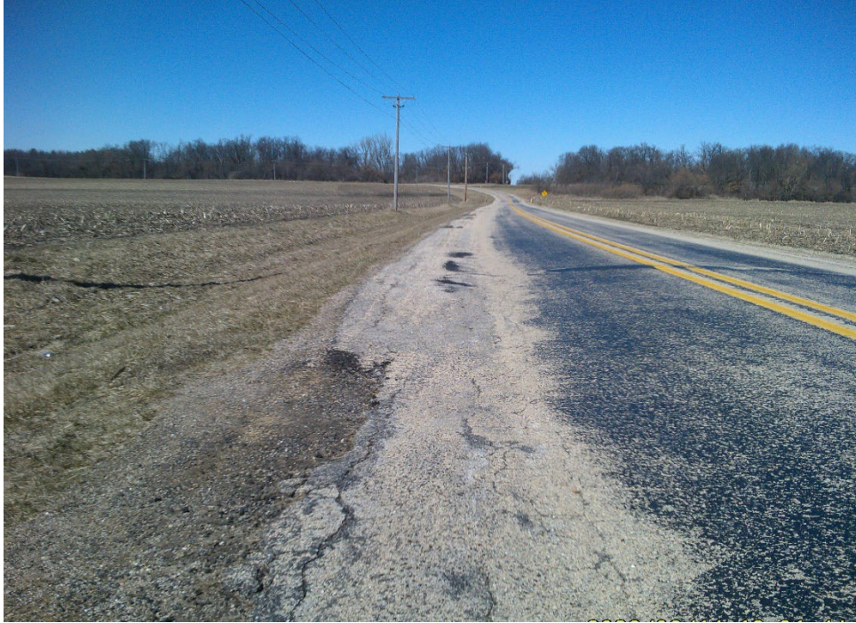
Sealcoat Rating 2 – Poor – Flushing, edge cracking and severe rutting
