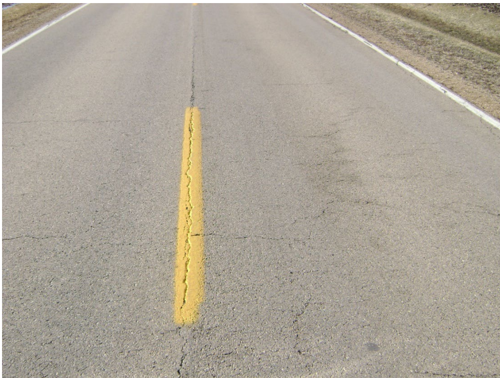
Asphalt Rating 6 – Good, transverse cracks less than 10 feet apart
