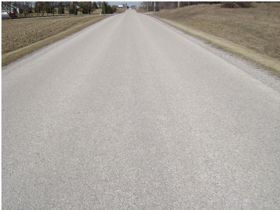
Sealcoat Rating 5 – Excellent – no issues/like new
