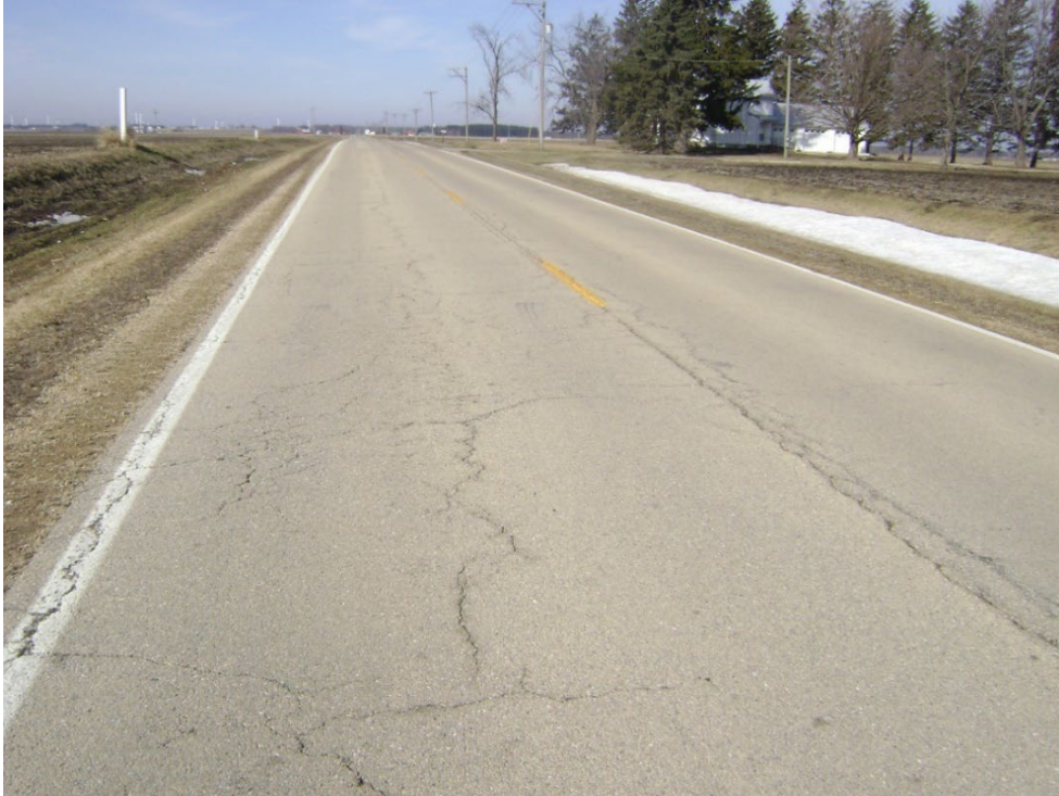
Asphalt Rating 5 – Fair, block cracking up to 50% of area
