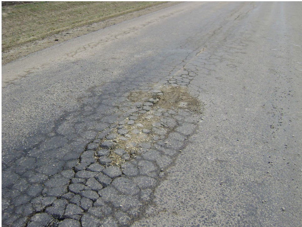
Sealcoat Rating 1 – Failed – loss of surface and mud is pumping into stone layer
