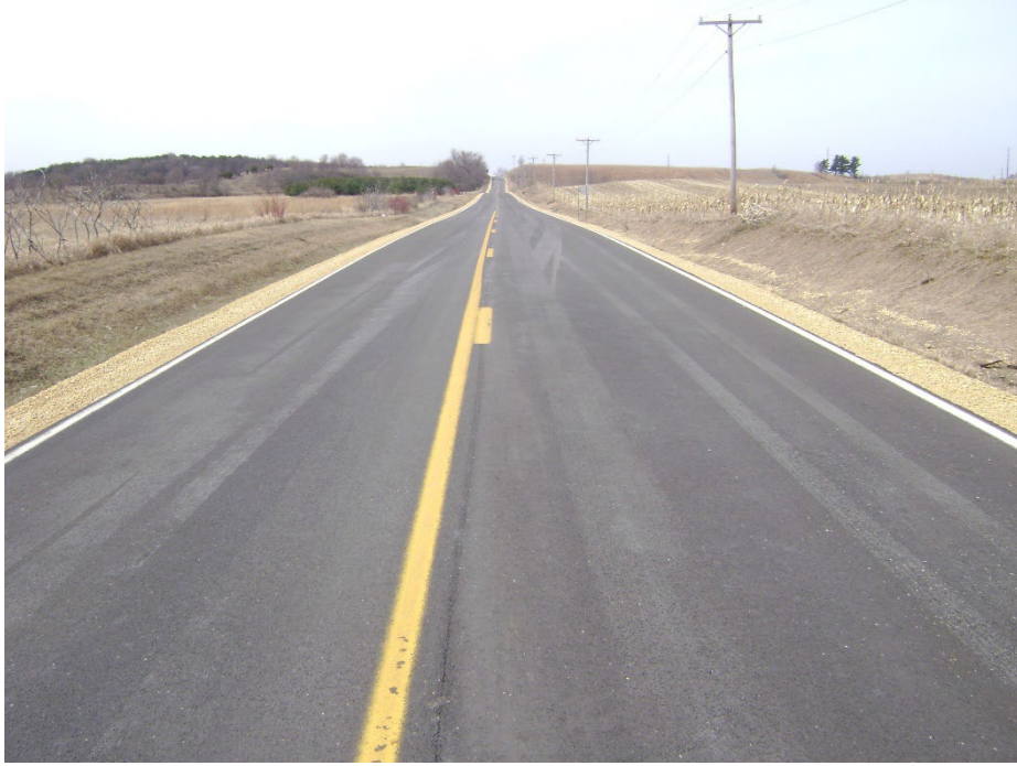
Asphalt Rating 9 – Excellent, recently placed HMA overlay
